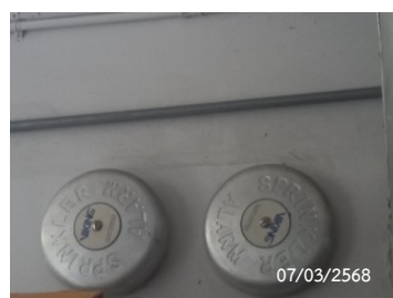
Sprinkler Fire Alarm
