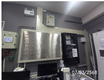
Graphic Annunciator Fire Alarm System
